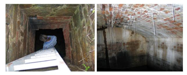
The second cistern is circular, about twelve feet in diameter, again with a very fine brick vault, and again about twelve feet deep – but this time with a lot of water in the bottom, since it has been incorporated into the surface water drainage system. We hope that the garage which was going to be put here will be moved so that both structures will be preserved.
