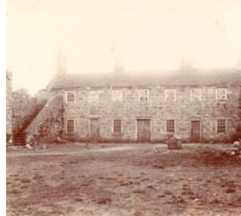
Officers' Quarters (South) fallen into disrepair. Photographed in 1892 © Guernsey Museums & Galleries
