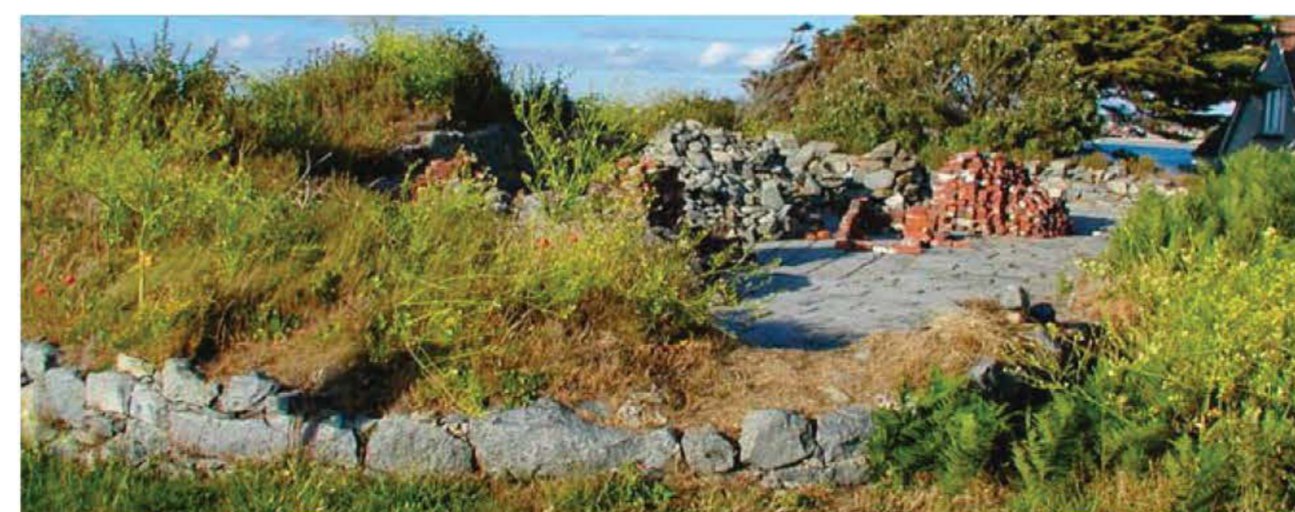
The Battery before restoration, 2007 Sandy Hamilton
